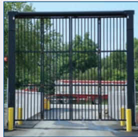
Top track gate
